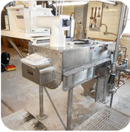
Campbell's Soup Manufacturing Plant, Napoleon OH
