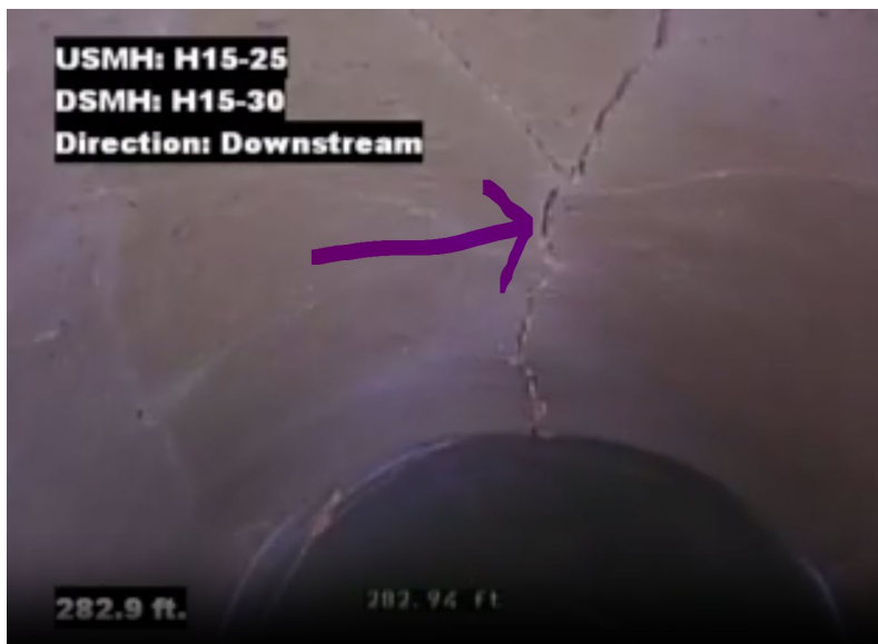
Cracked pipe
