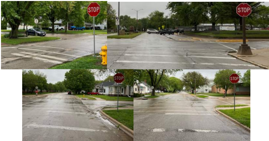
Exhibit 4: Painted Stop Bars near Webster City Middle School
