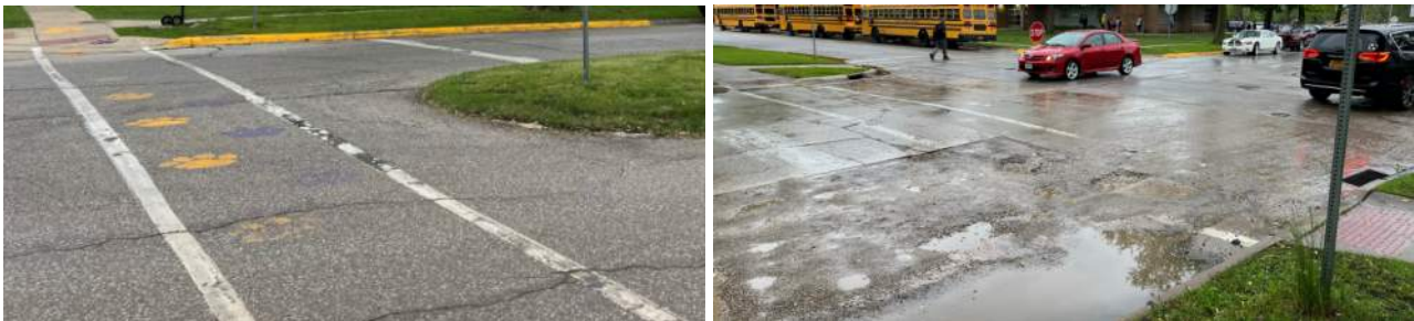
Exhibit 19: Crosswalk Pavement Markings
