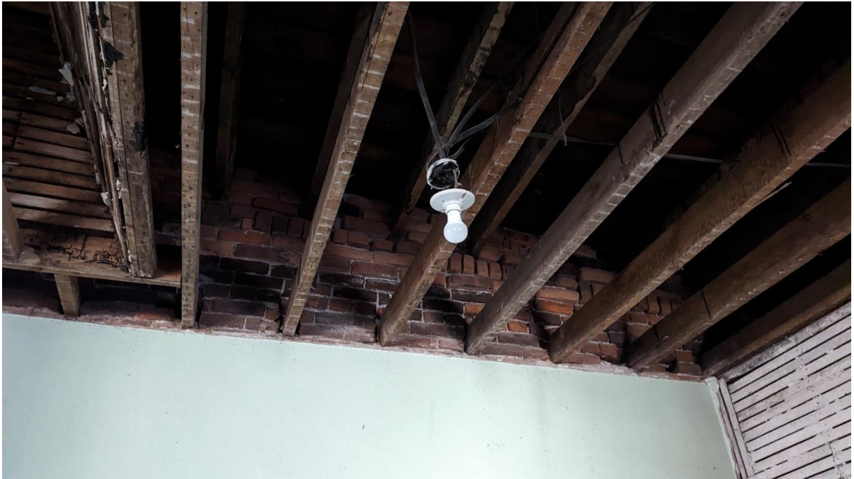
Photo 9. Deteriorated Mortar Joints along South Wall of 719
