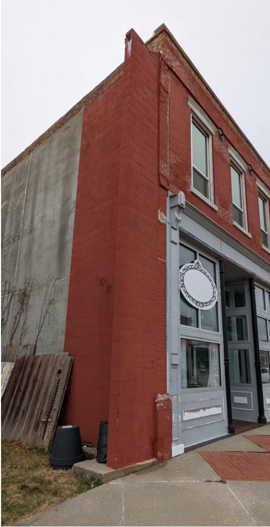
Photo 13 & 14. Example of a Shear Wall Laterally Reinforcing a Stand Alone Building
