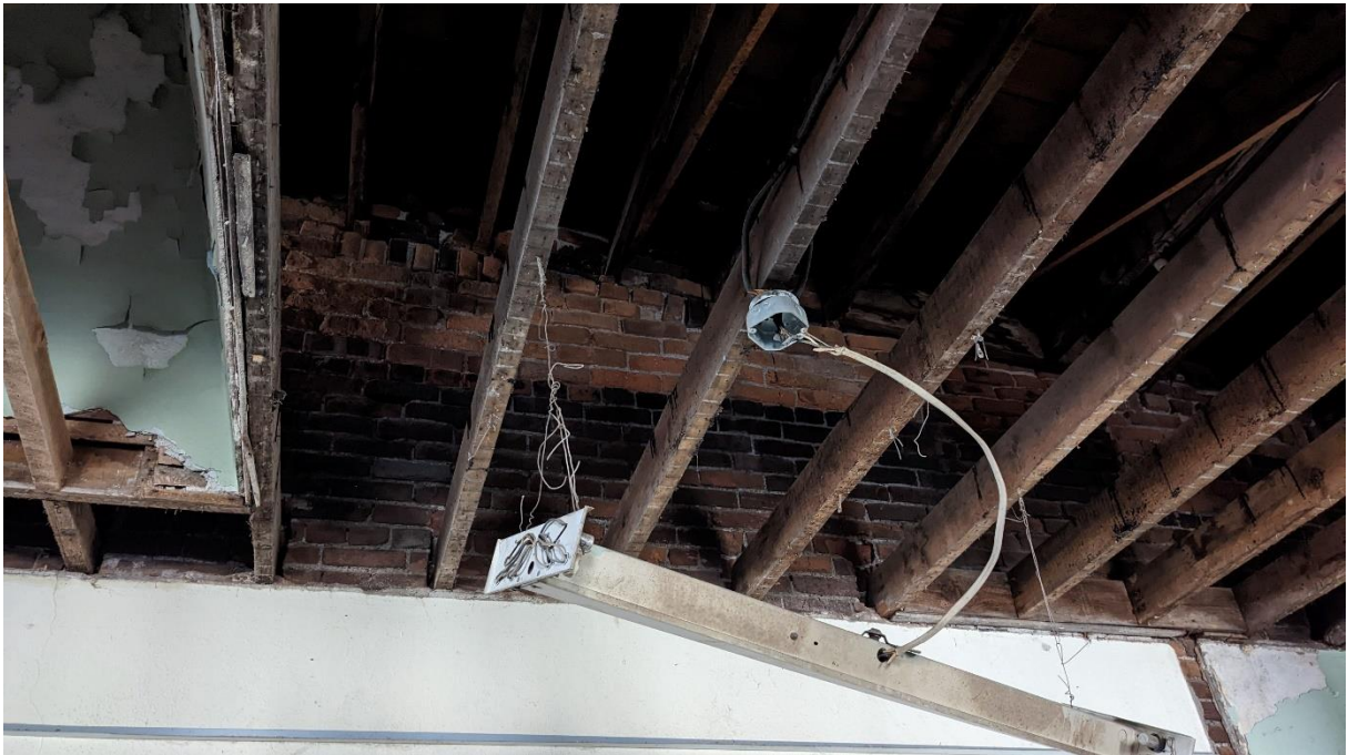
Photo 7. Deteriorated Mortar Joints along South Wall of 719
