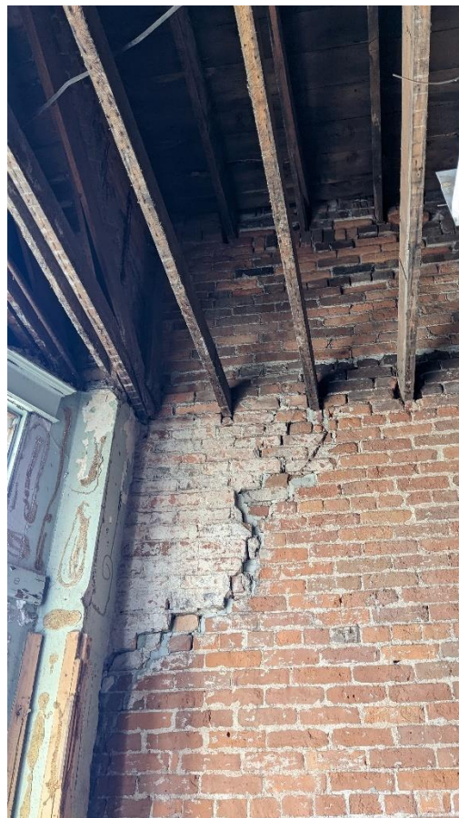
Photo 6. Previous repair and deteriorated Mortar Joins in SE corner of 719
