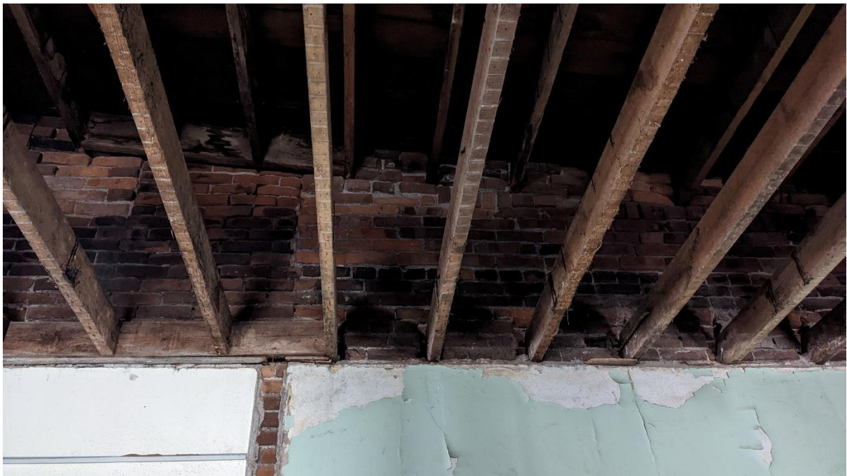
Photo 8. Deteriorated Mortar Joints along South Wall of 719
