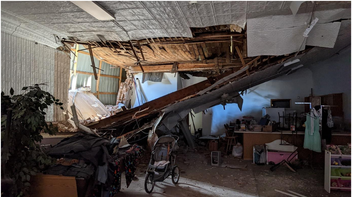
Photo 10. Collapsed Floor Framing in 721
