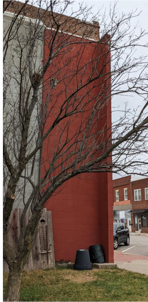
Photo 13 & 14. Example of a Shear Wall Laterally Reinforcing a Stand Alone Building
