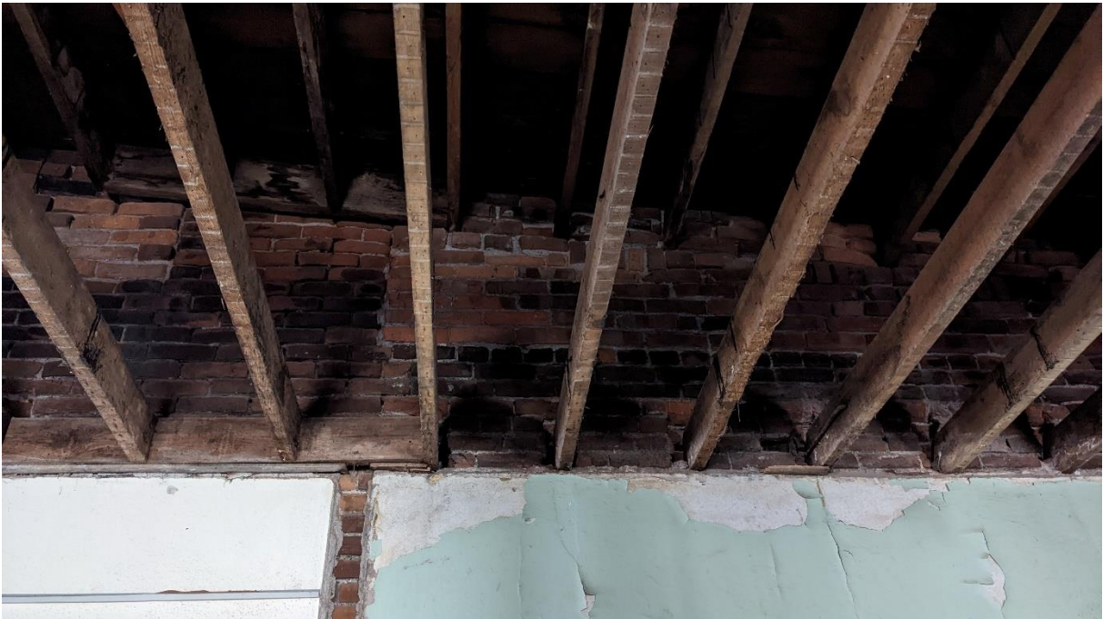
Photo 8. Deteriorated Mortar Joints along South Wall of 719
