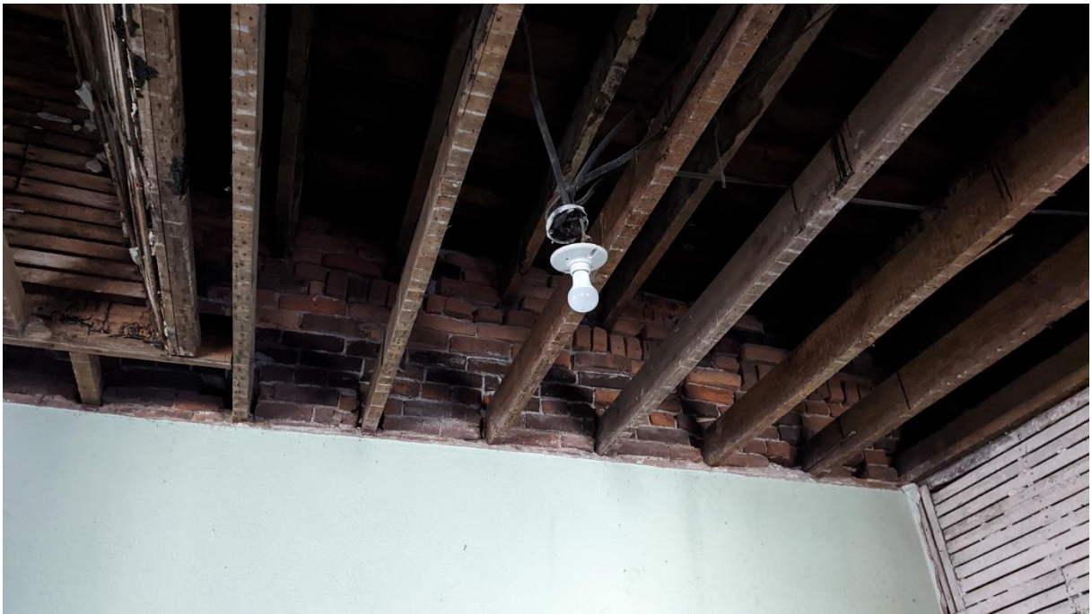
Photo 9. Deteriorated Mortar Joints along South Wall of 719
