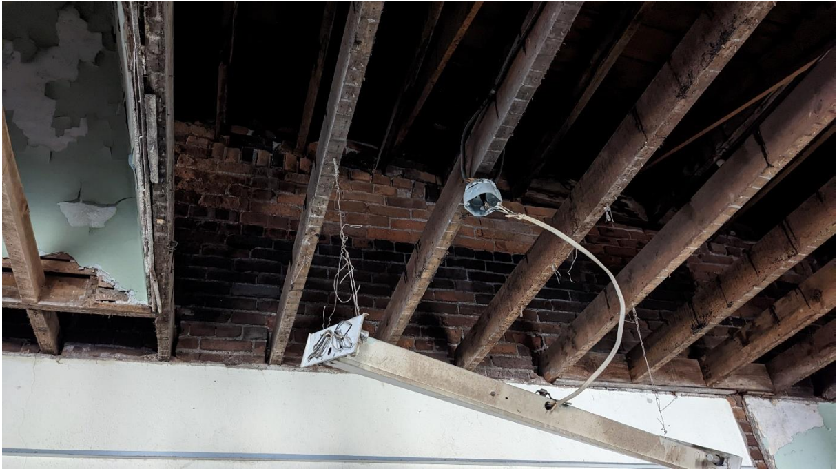
Photo 7. Deteriorated Mortar Joints along South Wall of 719
