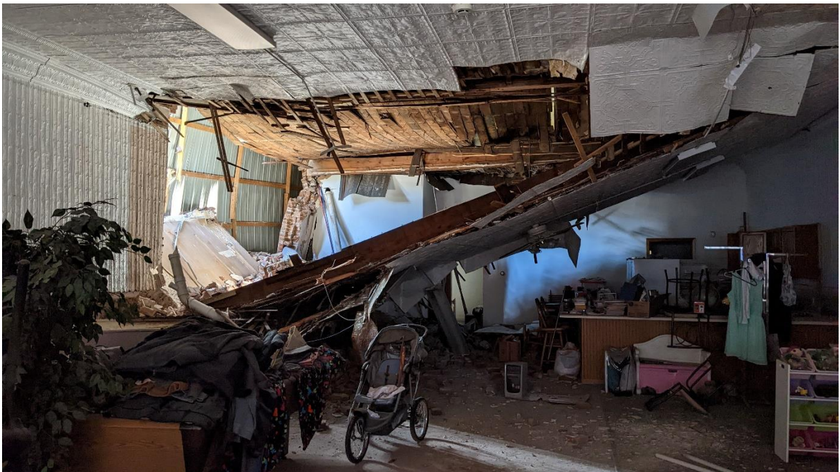
Photo 10. Collapsed Floor Framing in 721
