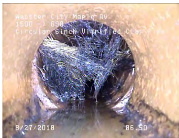
Roots growing into joints
