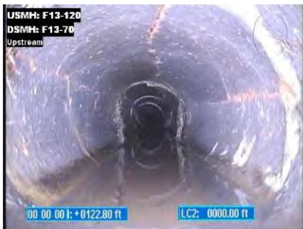
Cracks in Pipe
