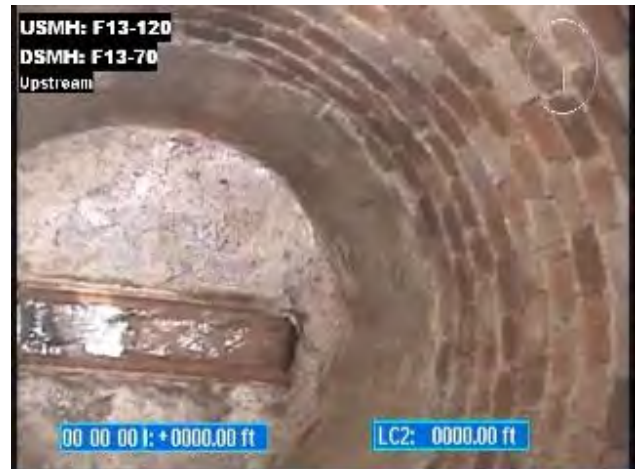
Deteriorating Brick MH
