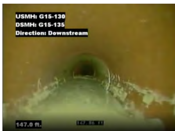
Build up of silt in bottom of pipe.
