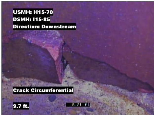
Cracks in Pipe
