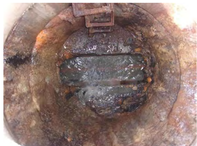
Deteriorating Pre-Cast MH
