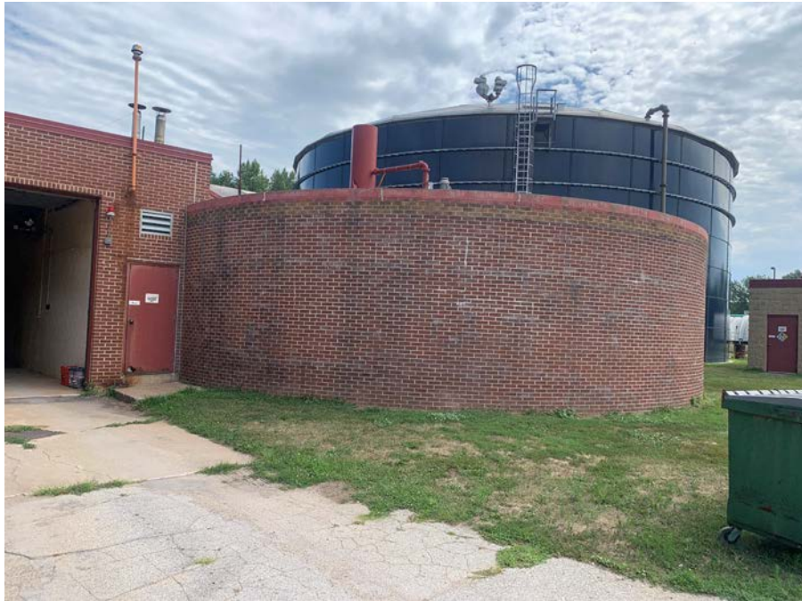
An anaerobic Digester (near) Biosolid Storage Tank (far)
