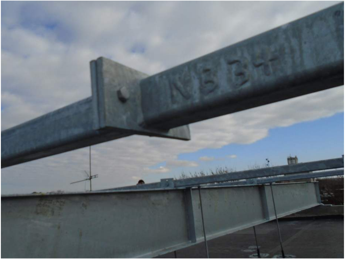
Photo 7: HSS tubes were to have drain holes installed.
