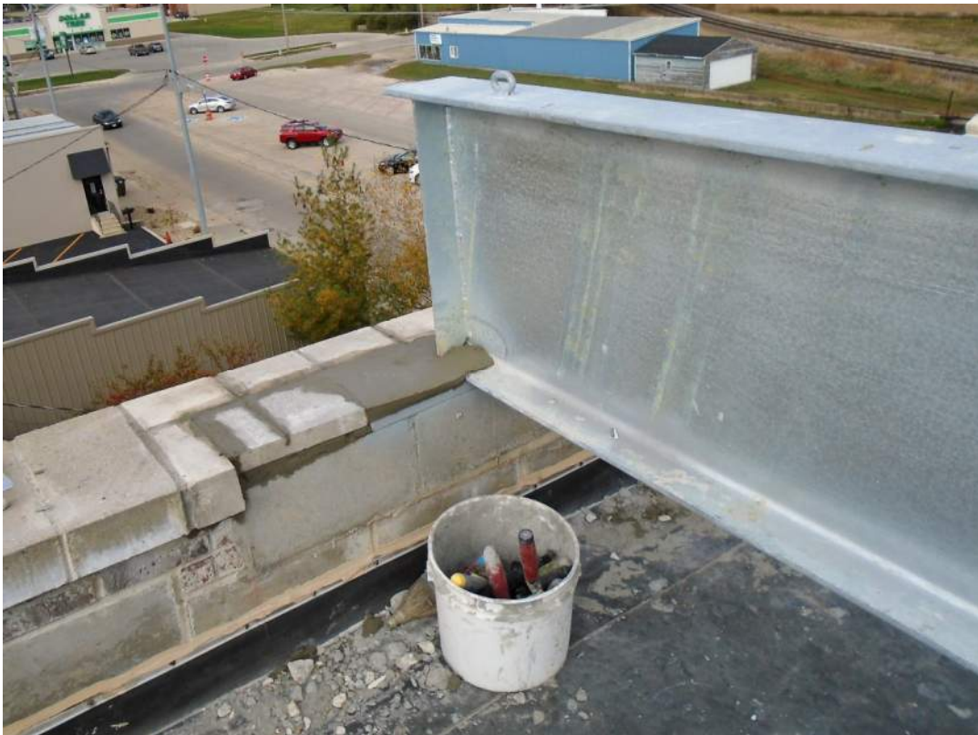
Photo 4: Beam at parapet with masonry installed
