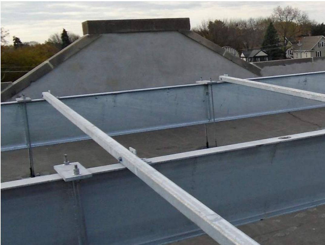
Photo 6: One nut missing from support rods
