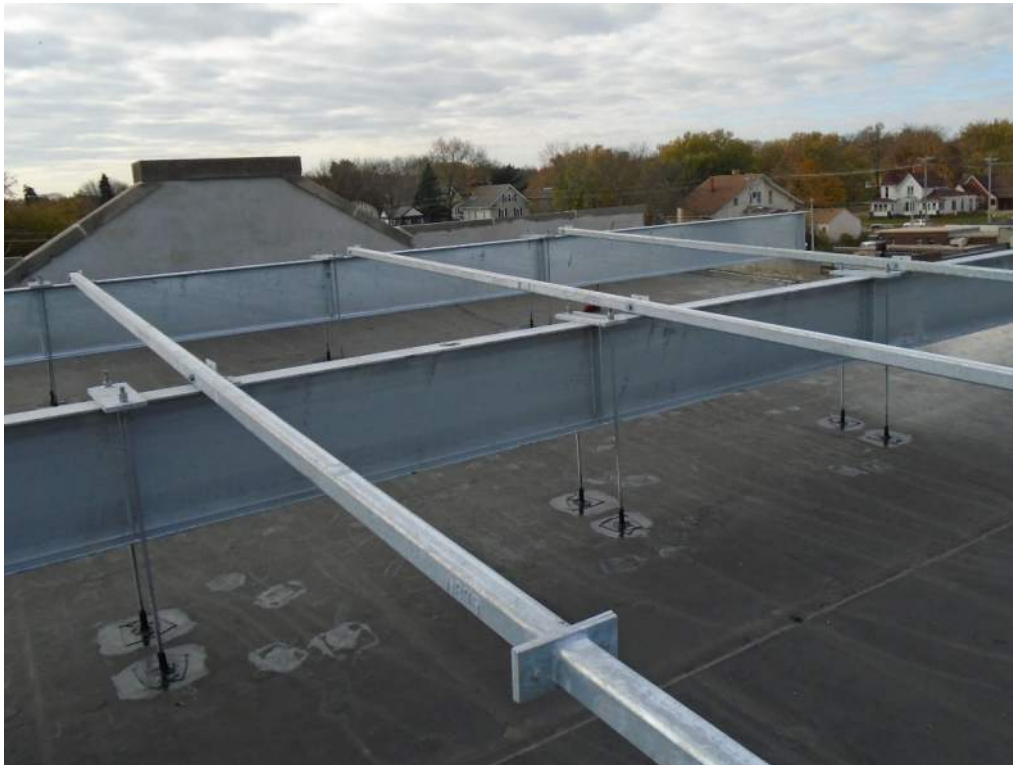
Photo 2: Support beams, rods and lateral bracing from outside building
