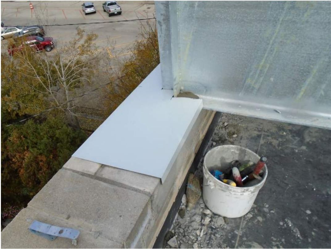
Photo 5: Flashing to be installed at beam ends – Architect and contractor working on sealant details
