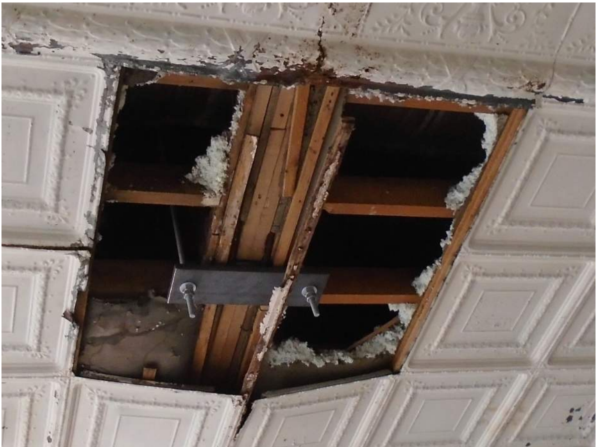
Photo 8: Closeup of hanger rods inside the building
