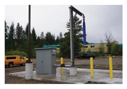
Top Loader quoted as an option. Piping is 3" Stainless Steel and support is painted steel.
