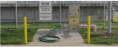
The FS-22 is ideal for reuse water and for locations that require a metered valve but not necessarily a backflow preventer. The FS-22 is freestanding and consists of the FS-20 model and a stainless steel enclosure to house additional valves.
