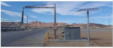
The FS-72 has all the features of the FS-43 and 63 models and additionally allows for greater customization for fill outlets (ie a bottom and overhead fill) for hauler trucks. It is compatible with up to 4" water supply pipes.
