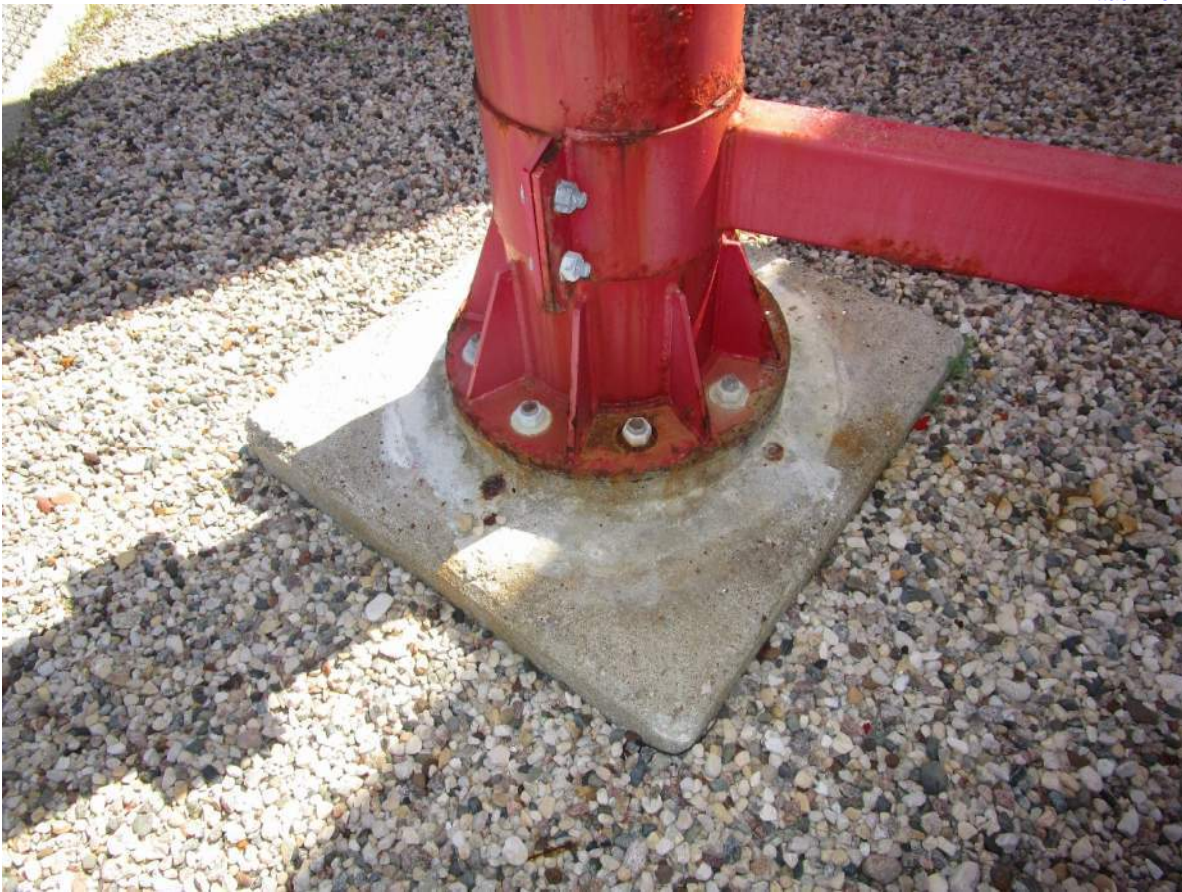
Photo 15: west slide support foundation
