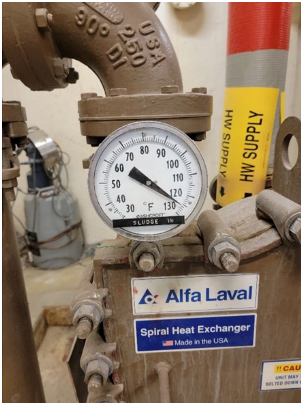
Figure 2: Heat exchanger should be around 95 degrees.
