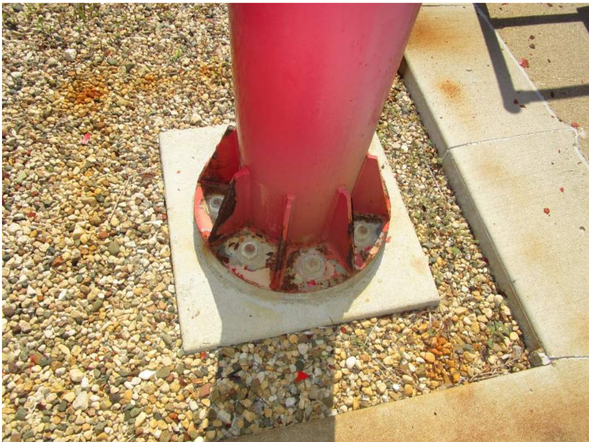
Photo 22: intermediate stair landing support foundation
