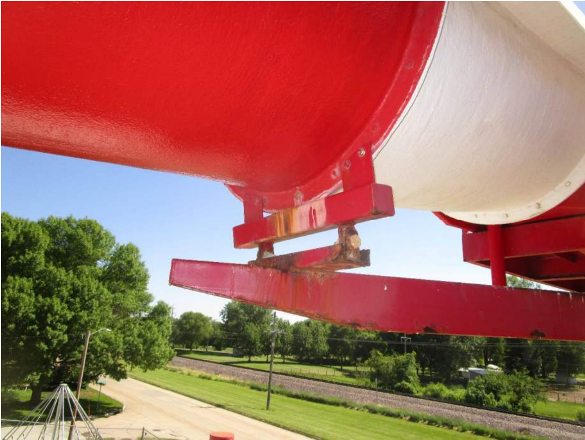
Photo 27: top landing slide support
