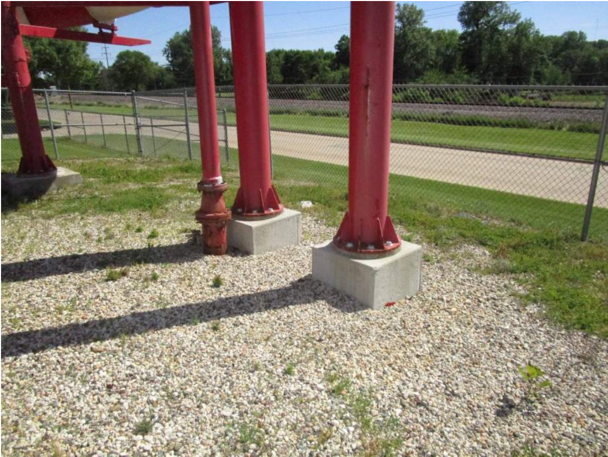
Photo 31: top stair landing support foundation and feed pipe
