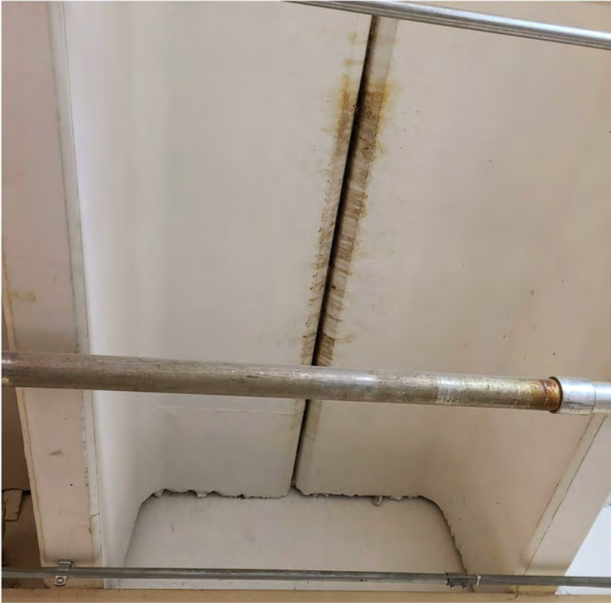
Seepage and staining at double tee joint.
