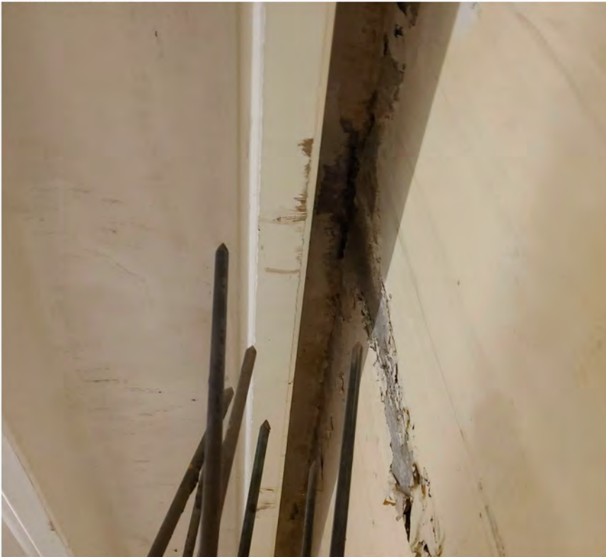
Delamination and spalling of concrete.
