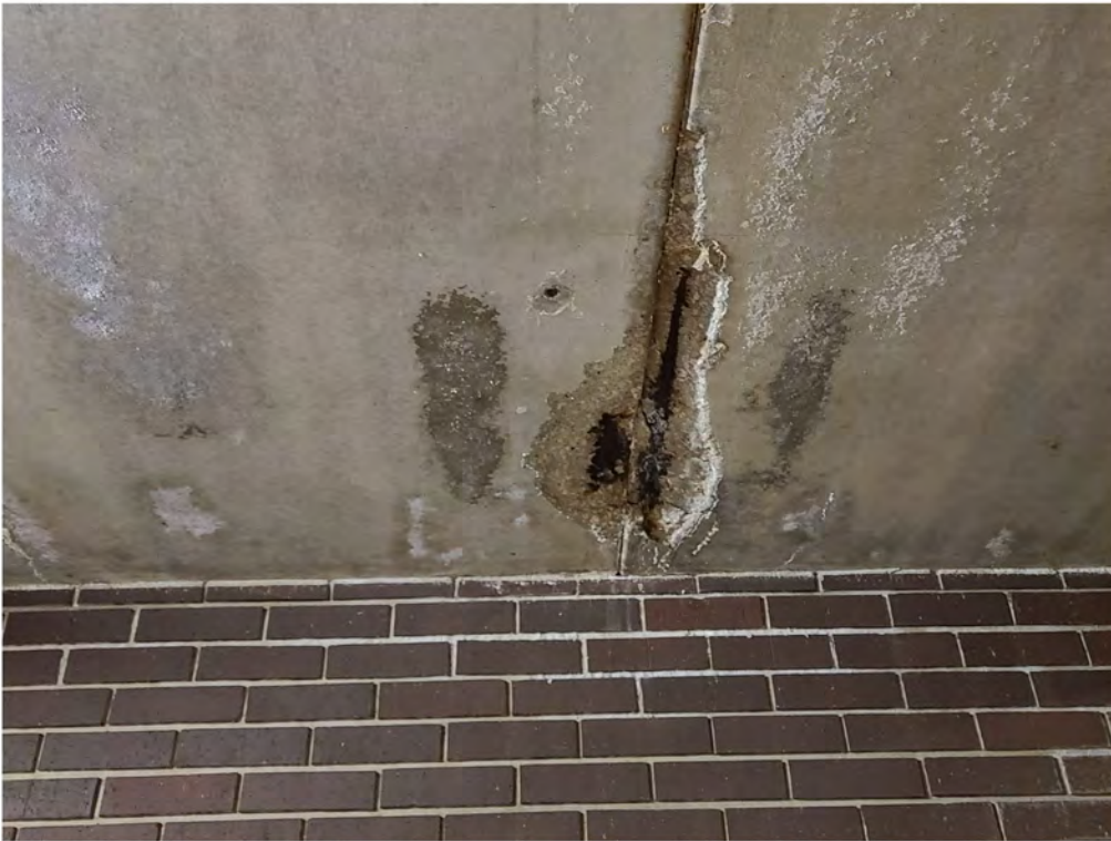
Spalling and cracking of concrete and pre-stressed strand rust.
