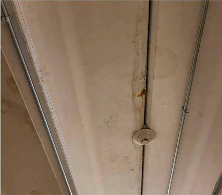
Delamination and cracking of concrete at double tee joint.
