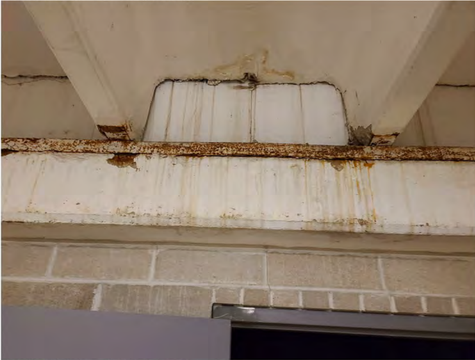
BB-2 (Right) and CC-1 (Left) Spalling of double tee stem. Rusting of bearing plate and spalling of beam.
