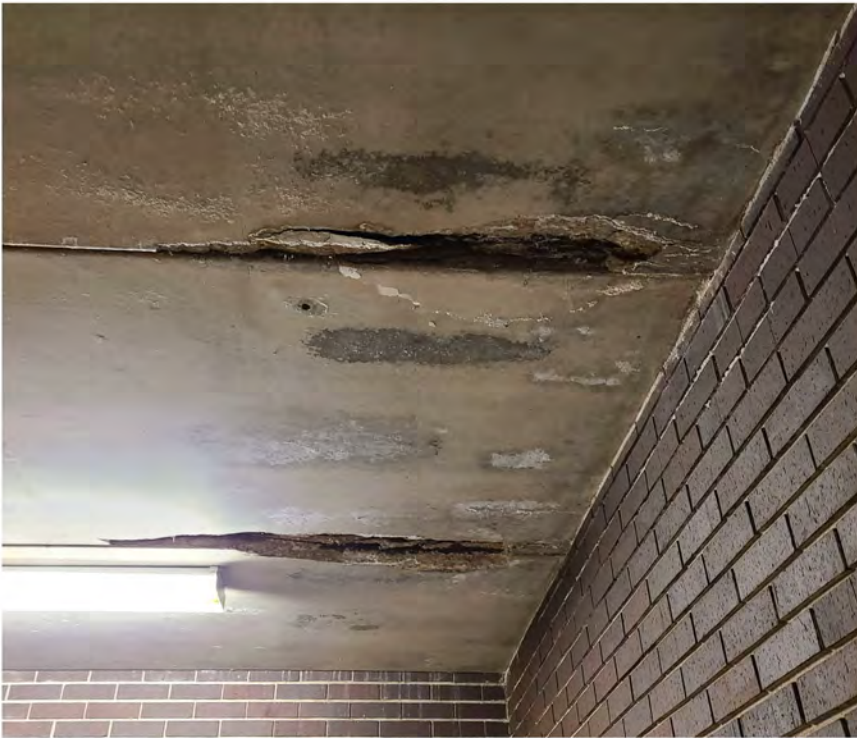
Spalling and cracking of concrete and pre-stressed strand rust.
