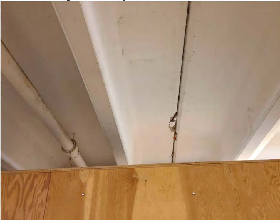
Localized cracking at double tee joint.
