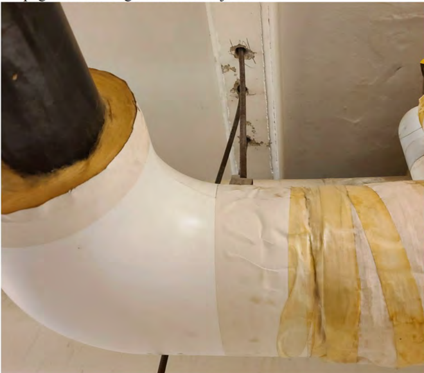
Seepage and staining at double tee joint.
