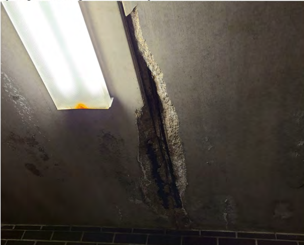
Delamination and spalling of concrete and pre-stressed strand rust.
