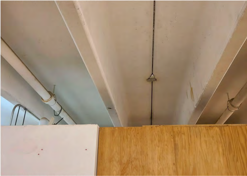
Localized cracking at double tee joint.
