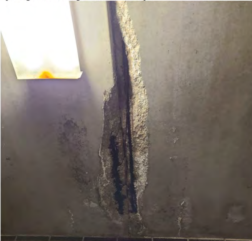
Spalling and cracking of concrete and pre-stressed strand rust with section loss.
