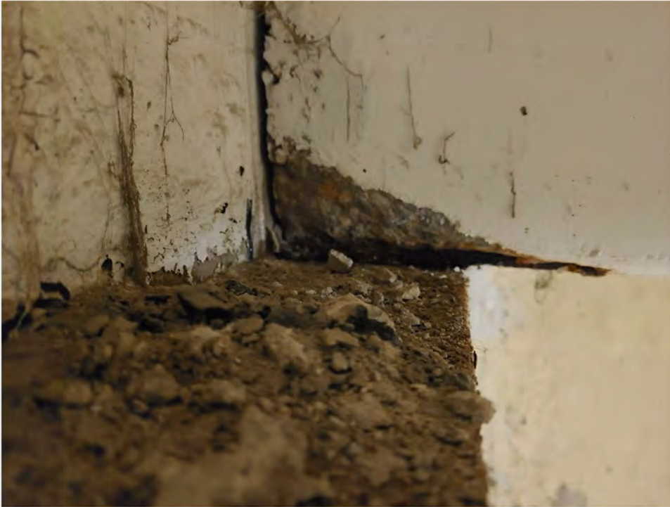
BB-1 Spalling of double tee stem.
