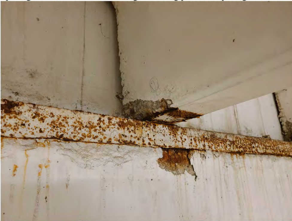
CC-1 Spalling of double tee stem. Rusting of bearing plate and spalling of beam.
