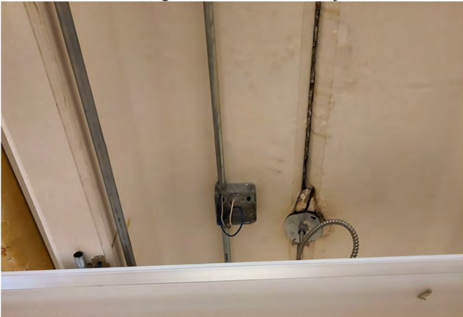
Localized concrete cracking at double tee joint.
