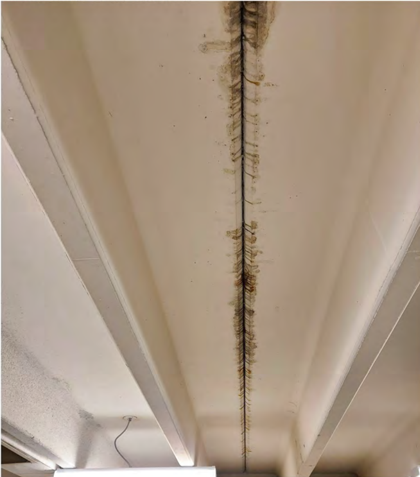
Seepage and staining at double tee joint.
