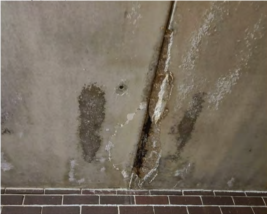
Spalling and cracking of concrete and pre-stressed strand rust.
