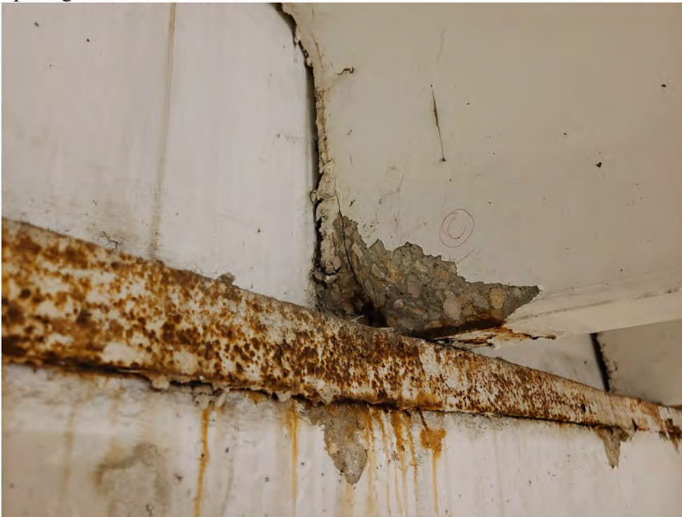
BB-2 Spalling of double tee stem. Rusting of bearing plate and spalling of beam.
