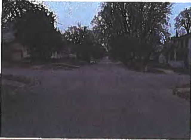
Prospect Street south leg, looking north at Boone Street
