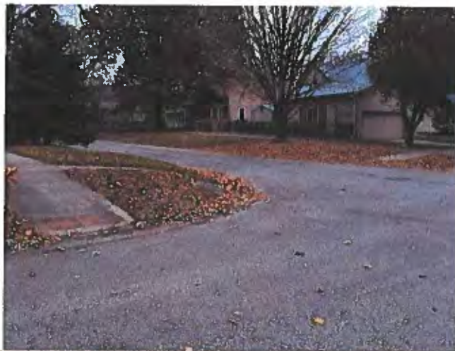
Prospect Street south leg, looking to northwest at Boone Street west leg
