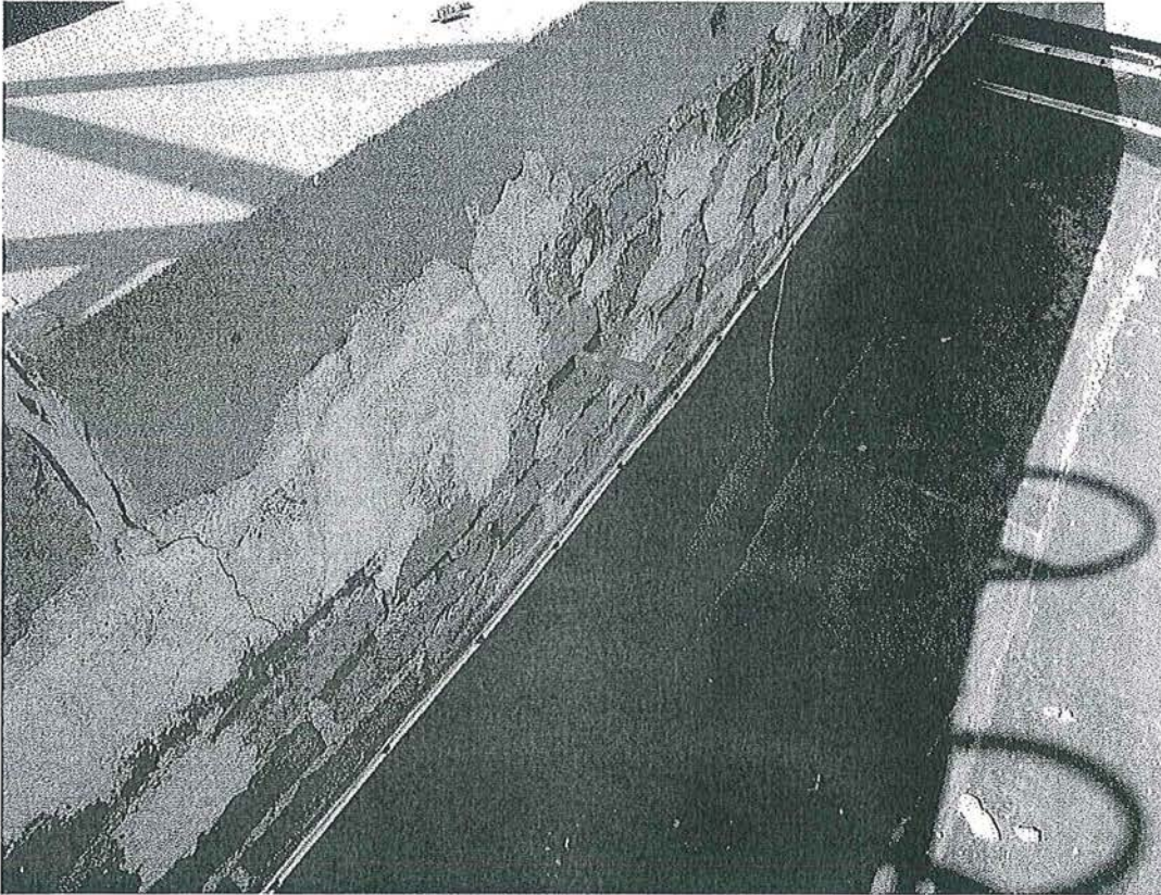
Photo 9: roof parapet on south side of building missing mortar sealant dried and cracked
