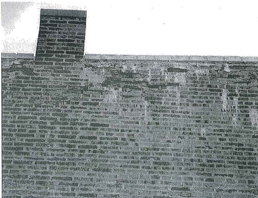
Photo 12: west wall missing mortar and brick faces
