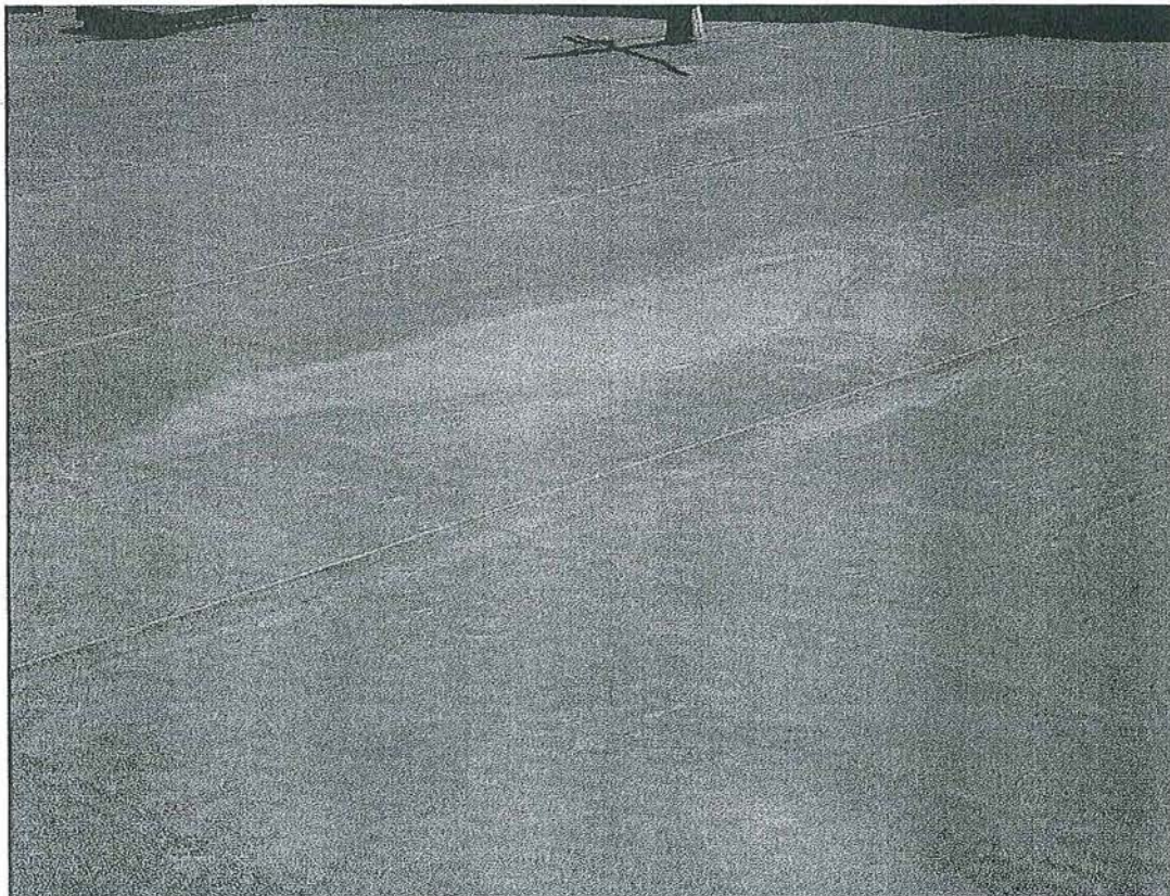
Photo 4: area of water ponding
