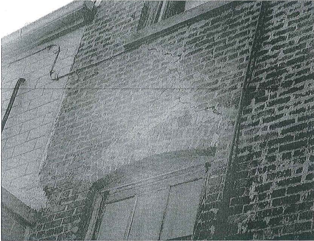
Photo 17: north wall stair step cracking
