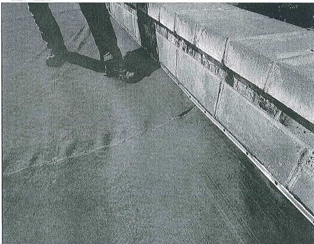
Photo 6: roof membrane hole where it appears the roof deck is below the membrane
