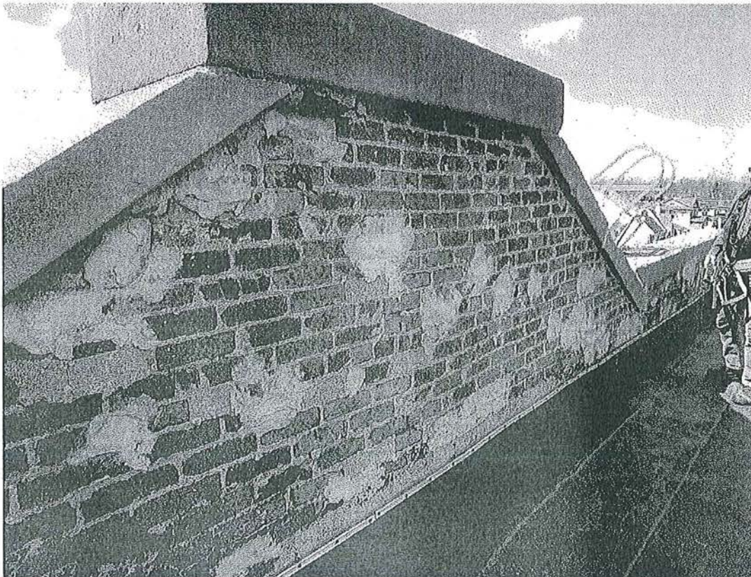
Photo 10: roof parapet on south side of building missing mortar and brick faces
